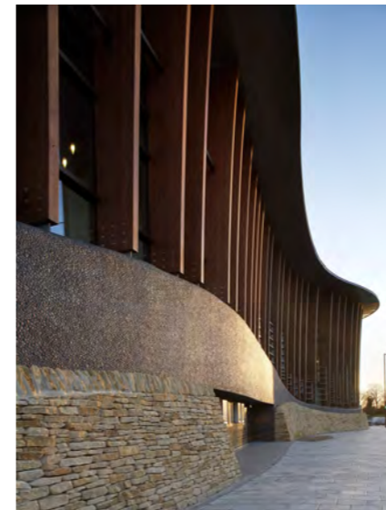
View of external timber frame and plinth
