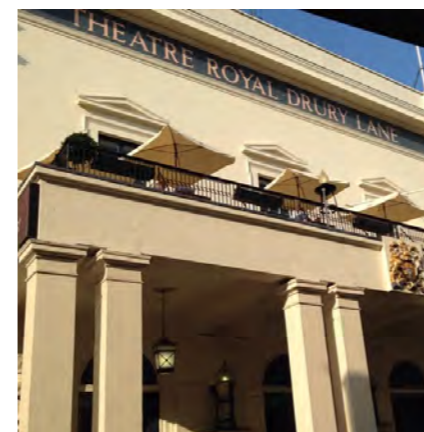
The completed terrace
